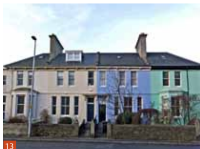
Fig 12 Beachtower, 6 Ralston Road, West Ferry, Dundee (1875). An early example of shuttered mass concrete used on a large domestic scale.
