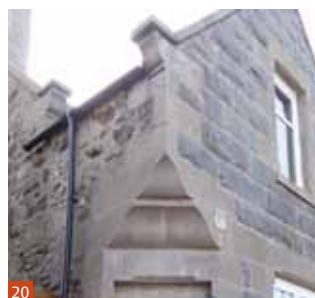
Fig 19 Winston House in Banff (1897). Painted precast concrete has been used to emulate stone quoins, dressings, margins and corniced chimney stacks within the squared rubble front elevation.
