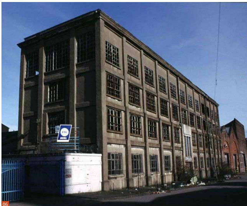
Fig 6 Sentinel Works, 61 Jessie Street, Glasgow (1903-4). An early ferro-concrete construction built on the Hennebique system. © Daniel Dubowitz
