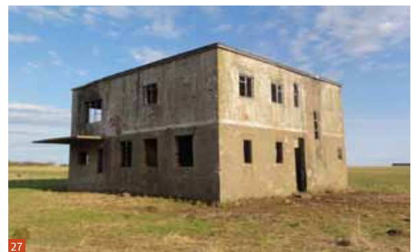
Fig 27 Control Tower, Boyndie Airfield, Banff (1943). Brick walls with reinforced concrete floors, roof and cantilevered balcony. Extensive corrosion of reinforcement has disrupted the ceiling of the intermediate floor.
