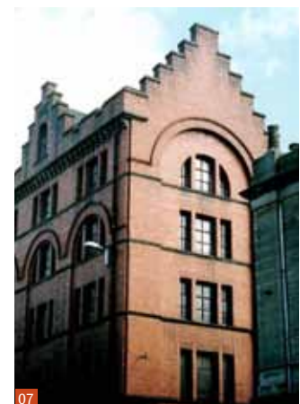
Fig 7 Watson's Bond, Seagate, Dundee (1907). Reinforced concrete frame using the Hennebique system and brick cladding. © Douglas MacKenzie
